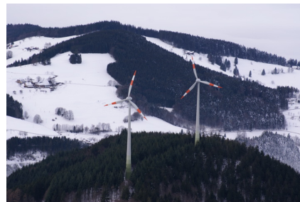
Figure 1. Wind power plant.
