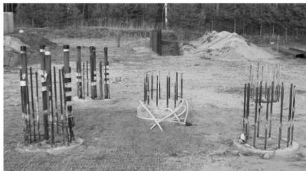
Figure 4. Pile Setting; the pile in the centre of the picture is equipped with fibre optic sensors.
