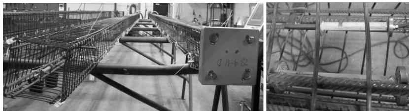
*Figure 8. Left: Reinforcement cages of Pile 1 (left cage) and the upper pile of Pile 2 (right cage), right: EFPI sensor (upper sensor) and reference sensor (lower sensor).*
