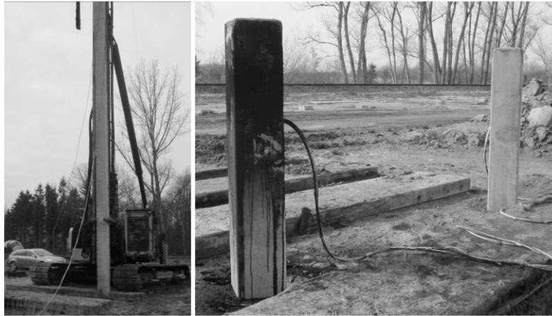
*Figure 9. Left: Driving of pile 1, right: precast piles after driving.*
