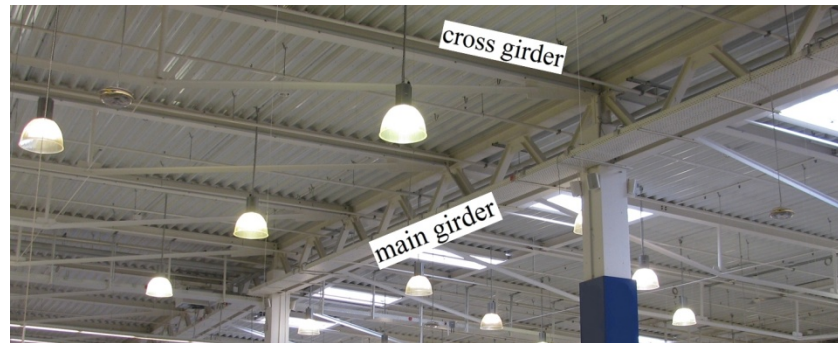
Figure 5. Bottom view of the roof structure.
