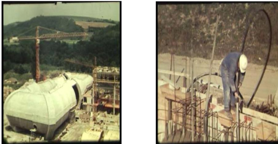
Figure 1. Construction (left: Wind-Tunnel overview, right: post-tension setup)
