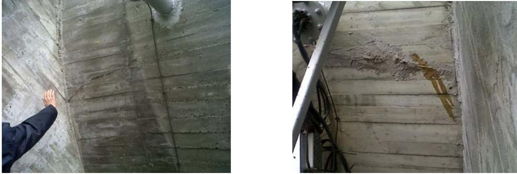
Figure 2. Visible microcracks causing air leaks when pressurizing (left: resin repair).
