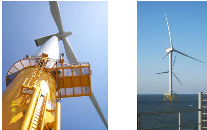
Figure 1. Typical Monopile Wind Turbine (left) and Mini Jacket type Wind Turbine (right).
