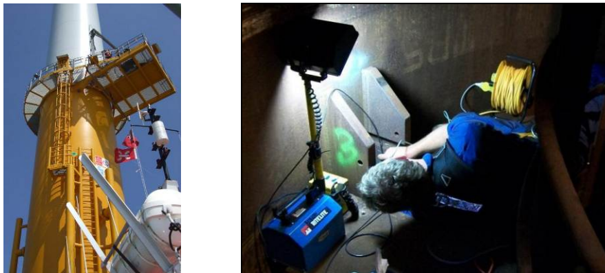
Figure 4. External access from workboat (left) and awkward installation conditions (right).
