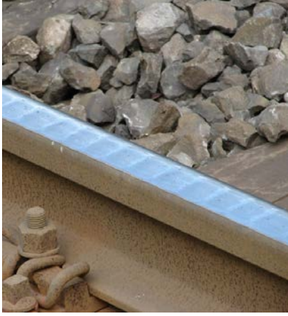
Figure 4. Rail corrugation example and its approach in numerical simulation.
